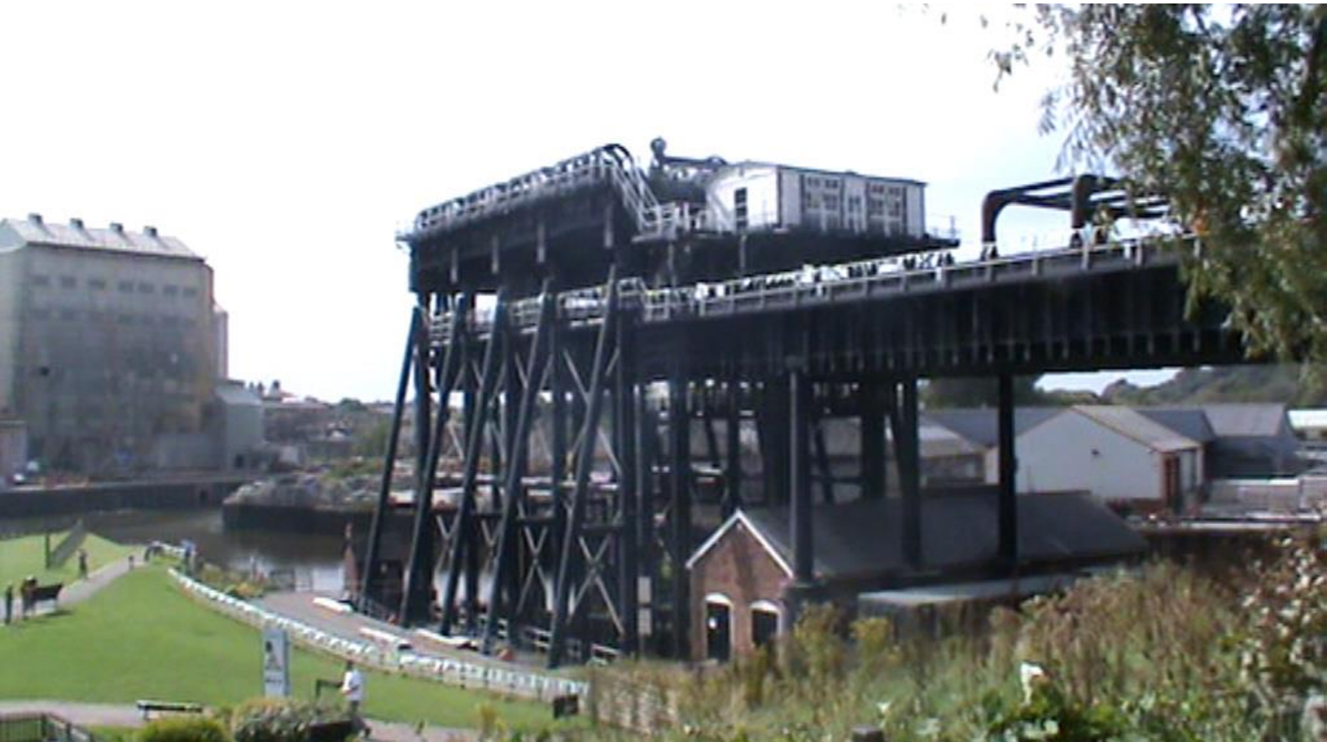
Anderton Boat Lift linking The Weaver Navigation and the Trent & Mersey Canal
